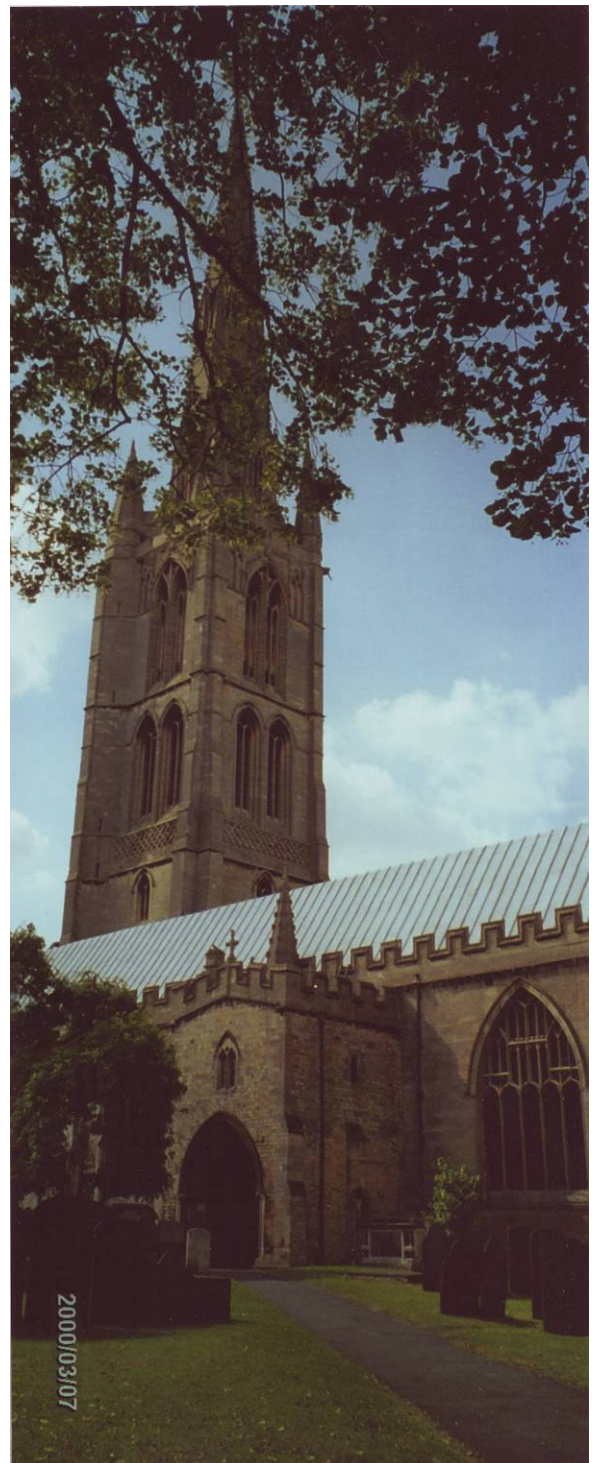
St Wulfram's Church, South Porch
